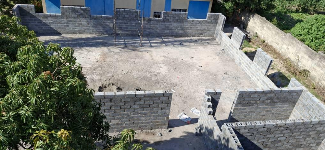
Figure 15: Wall erection
