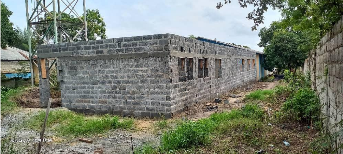
Figure 16: Completed ring beam construction
