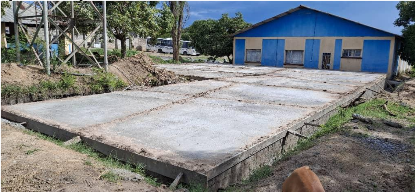
Figure 14: Slab curing
