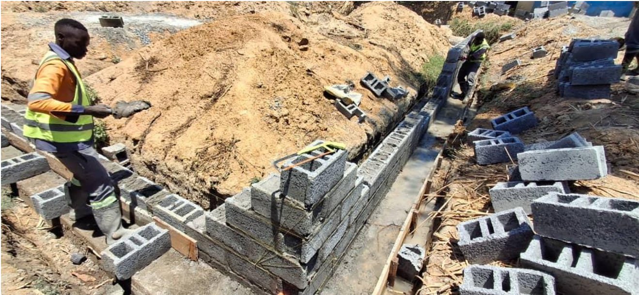
Figure 12: Foundation walls construction
