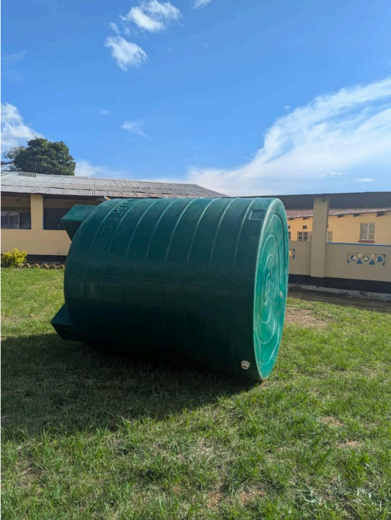
NEW WATER TANK
