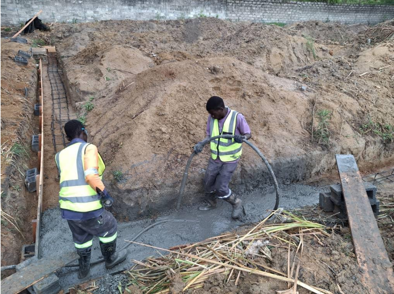
Figure 11: Pouring Concrete
