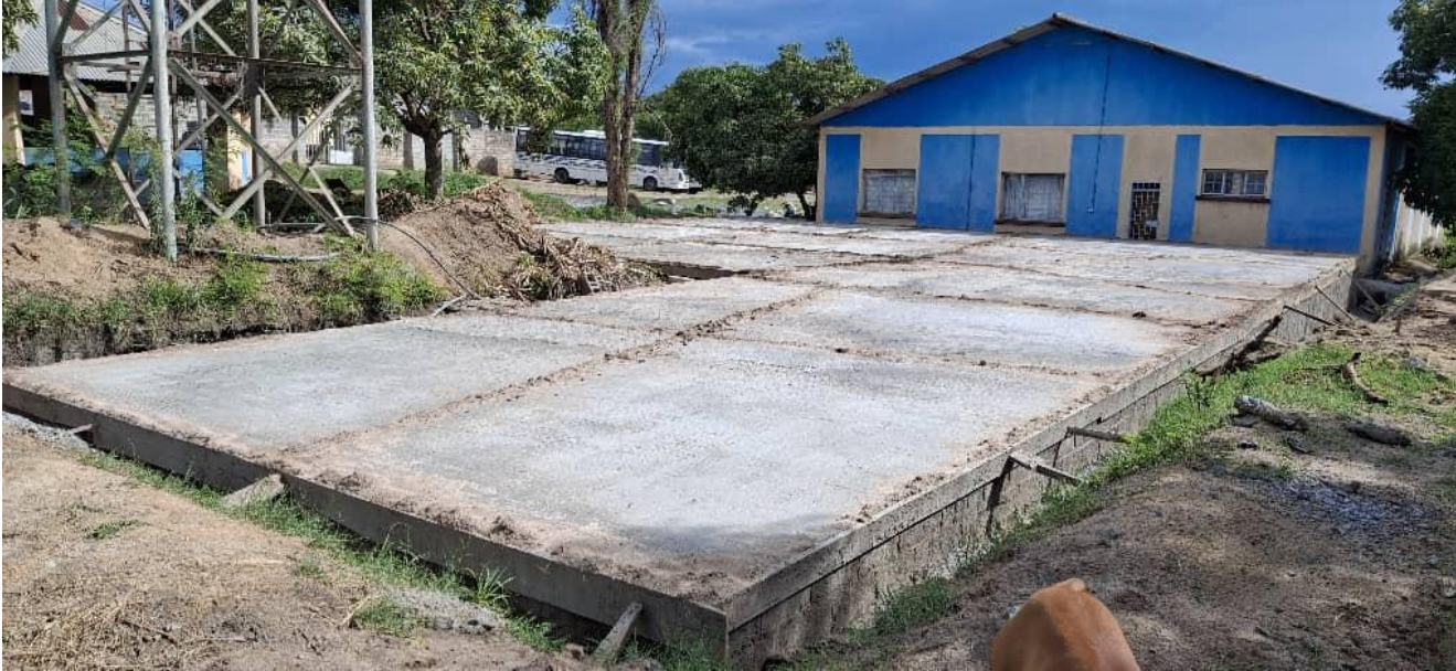
Figure 14: Slab curing
