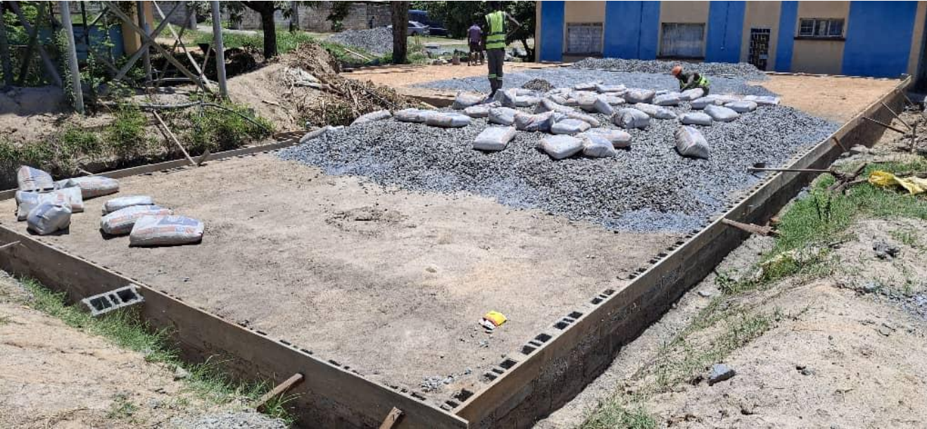
Figure 13: Construction of slab
