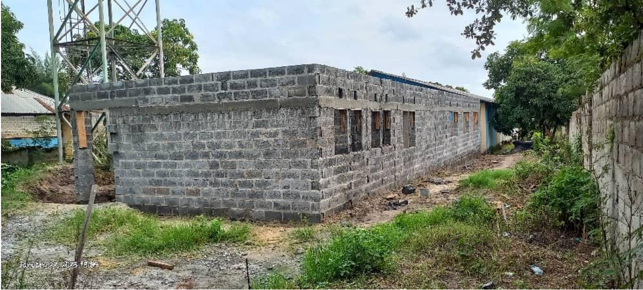
Figure 16: Completed ring beam construction
